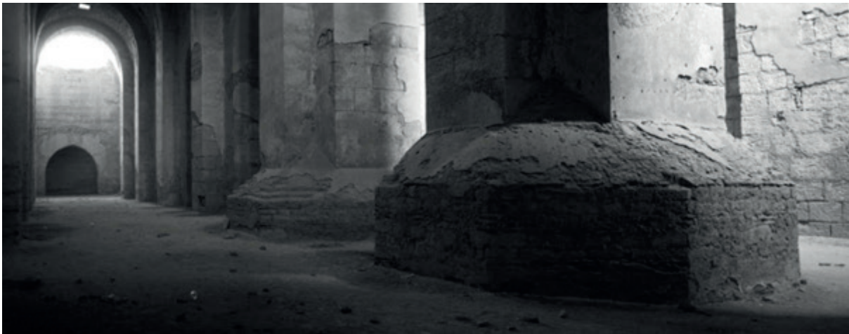
Figure 13. The "large cistern" in Resafa, Syria. It was filled by channeling periodical floods from a wadi west of the city into the cisterns and had a capacity of ~18,000m 3 .
