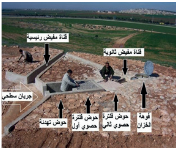
Building the underground cistern.
