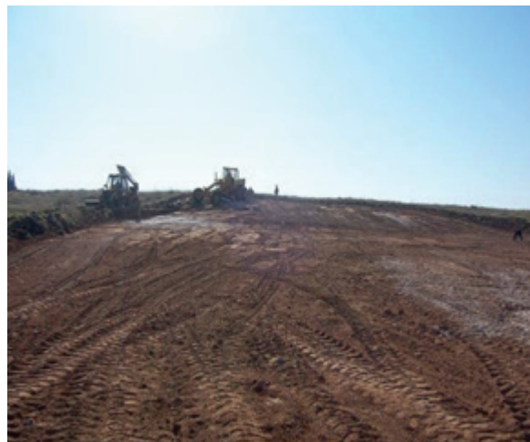
Preparing the site #2.
