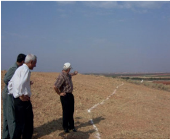
Preparing the contour lines in the site #1.
